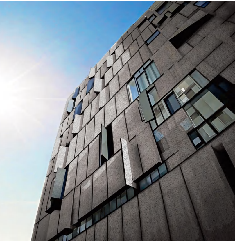
eSolarFacade Stone Ridged Ash Grey 2300mmX570mm (customized size) 50W/m² -120W /m²
