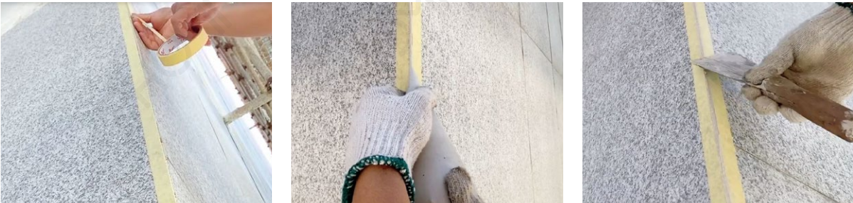
1.Paste masking paper 2.Caulk 3.Grout
