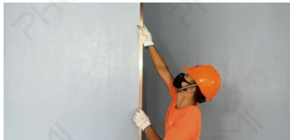
2.Stick the metal edge strips in external angle
