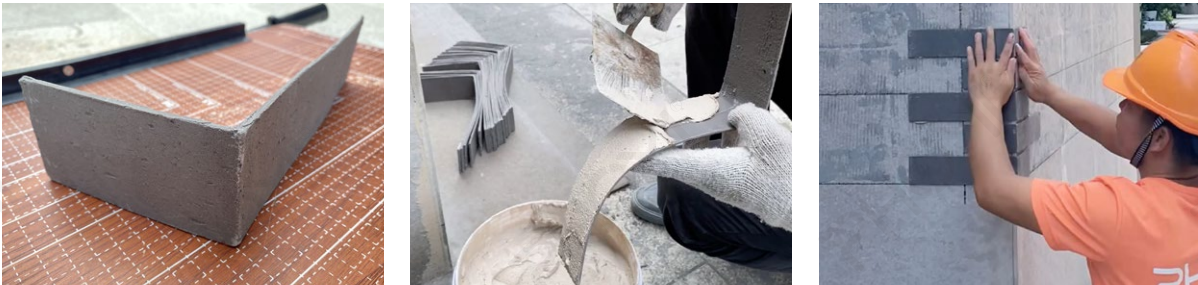
1.Corner brick 2.Scrape pulp 3.Paste
