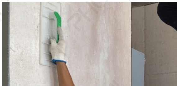
5.Compaction with board and guiding ruler
