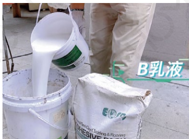
1.pour emulsion B into the barrel
