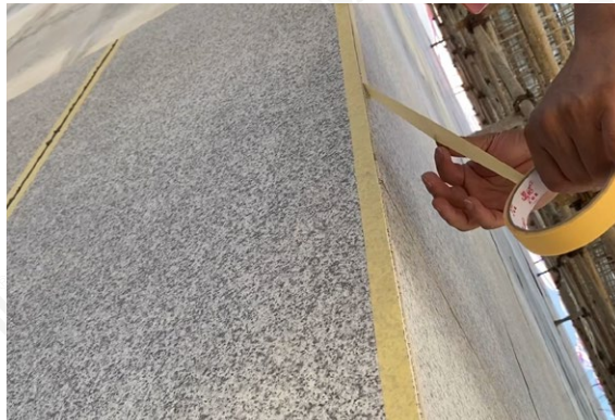
1. Paste masking paper along the external angle
