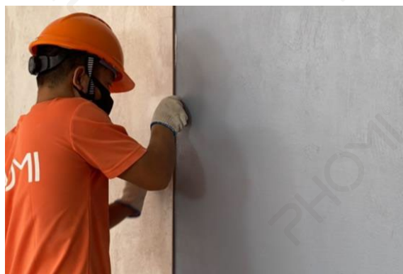
1. After pasting one side of the product, Compaction the decorative seam strip along the edge of the product tightly.
