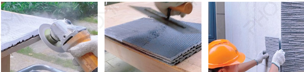
1.Grinding to make 45° chamfer 2.Scraping Paste 3.Paste
